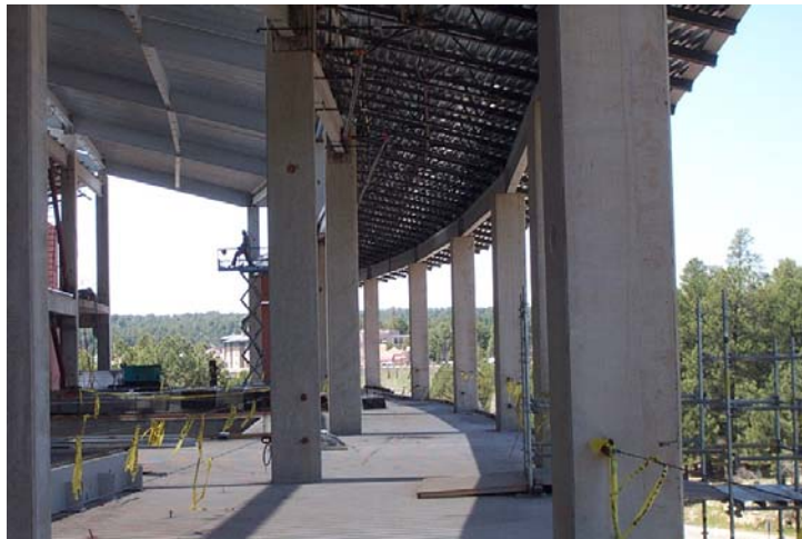
Figure 24 – CBA under construction
