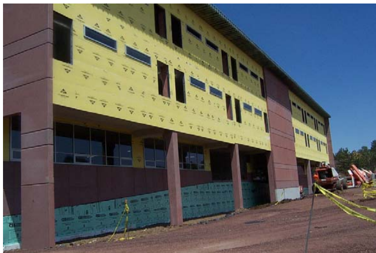
Figure 16 – Walkway during construction
